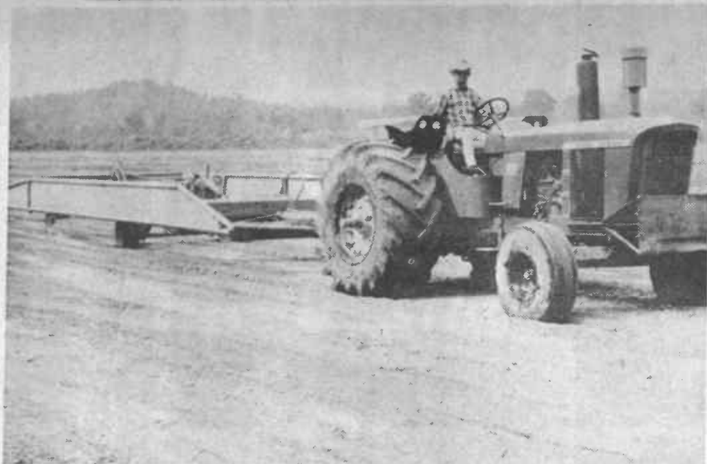
THE LAND PLANE — This machine is used in the final stages of drainage land-grading on the Frank Brinkley
